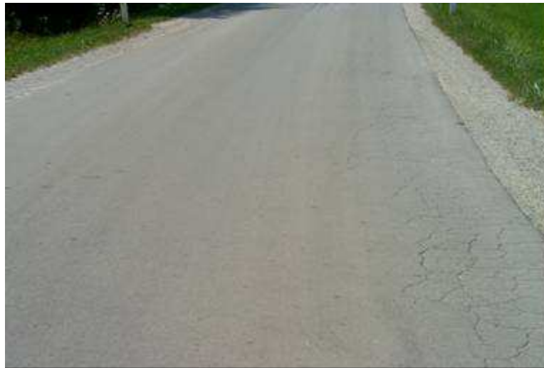
Picture 1 Example of a pavement suitable for rehabilitation by surface dressing
