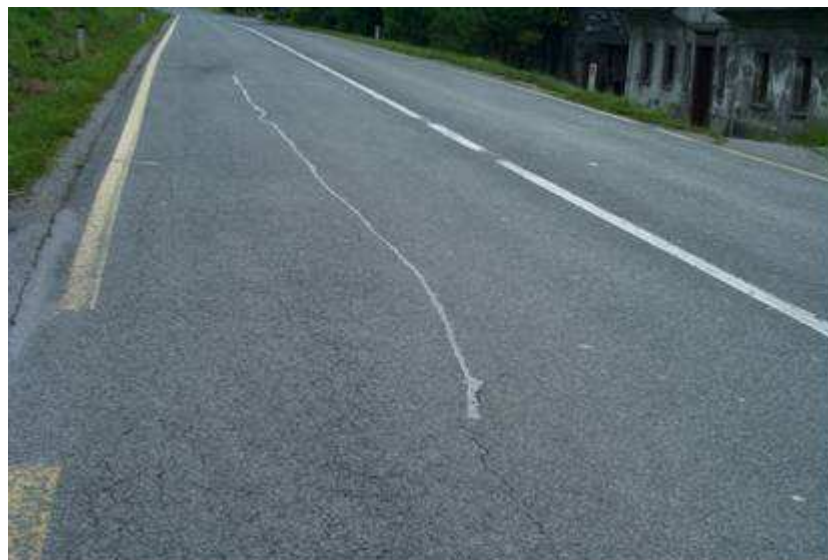
Picture 3 Example of pavement suitable for upgrade by asphalt layers
