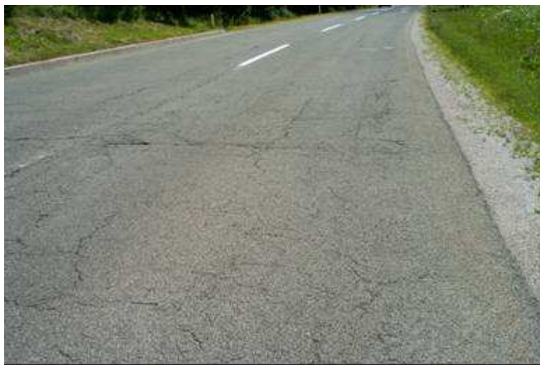
Picture 2 Example of a pavement suitable for overlaying with Asphalt Concrete – AC surf
